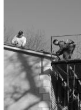
Ken Stacey and Nick Savini (above) nail down new roofing material after Bob Leonard and John Kreatz (below) removed the balustrade in sections.
