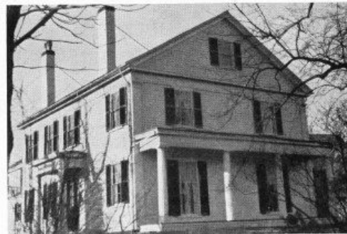
FIG. 4. DAY HOUSE 38 Kirkland St. Greek Revival, with one story porch. About 1840.
