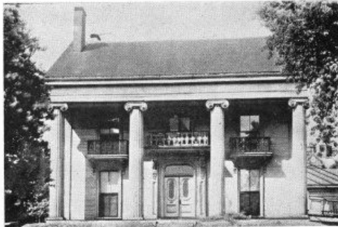
FIG. 3. ANONYMOUS (Demolished) Massachusetts Ave., corner of Dana St. Greek Revival, no gable. About 1850. (Photograph by Lois L. Howe.)
